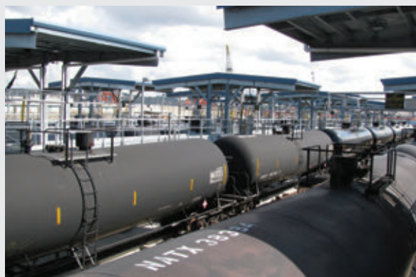
Rail loading facility.
