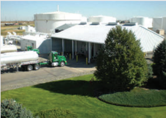
Truck loading facility.
